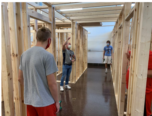
Residential Wiring Instructor Matt Dawson details the strength needed in a supporting structure for proper installation of a ceiling fan and other overhead electrical fixtures.
